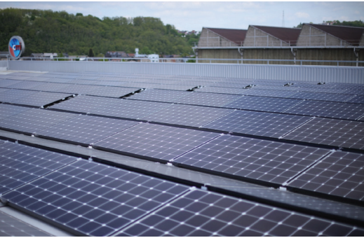
Figure 2. PV panels, part of CMI Energy's MiRIS project. MiRIS will be integrated with the CMI Group's international headquarters complex, allow its engineers to perform detailed analysis of renewable integration with energy storage. Source: CMI Energy
