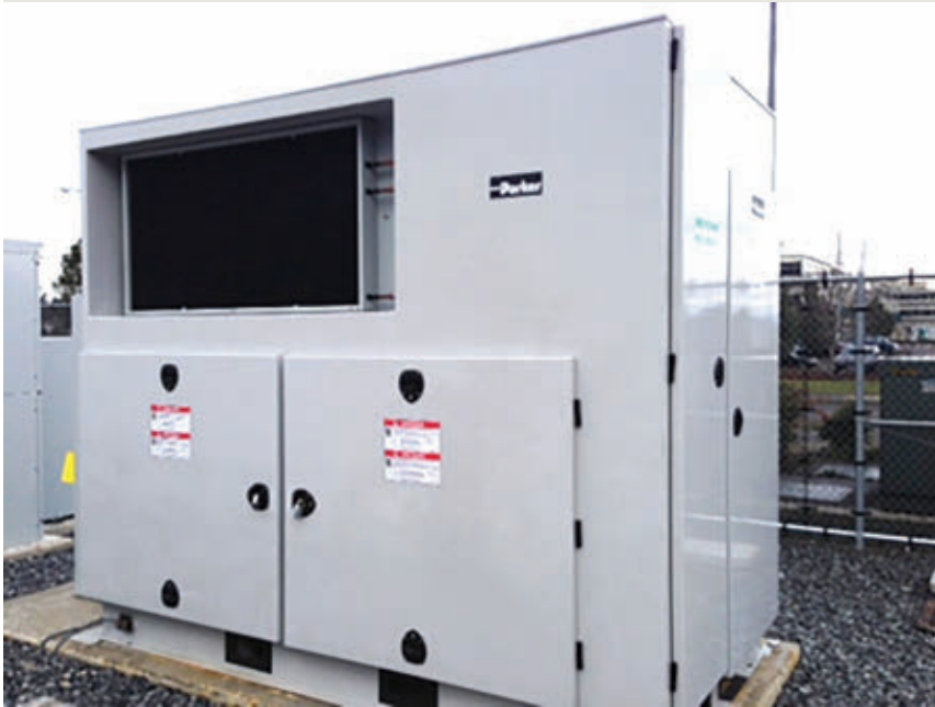
The Parker 890GTS/GTB is used on solar as well as BESS energy storage systems. The enclosure houses the PCS and thermal management systems for a BESS size up to 2 MW.
