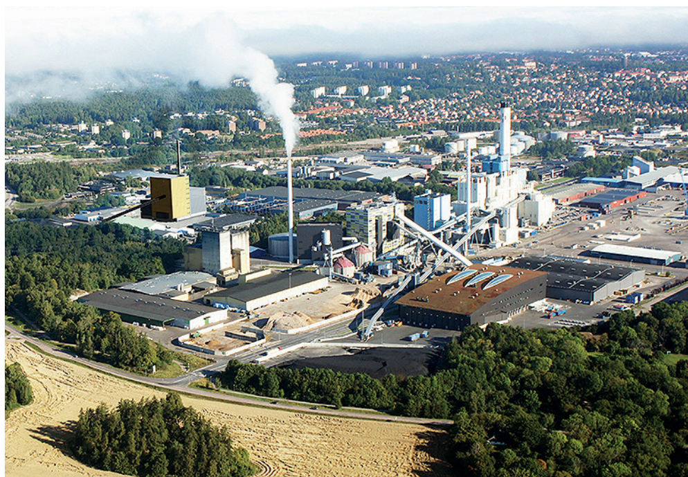
(Above) Photo rendering showing the siting of Mälarenergi’s Block 7 biomass-fired CHP at its Västerås facility. The order, a 152 MWth CFB, is the first under SHI FW (image courtesy Scheiwiller Svensson Arkitektkontor AB). (Left) The new 75 MWe Summit Handa Power Corp. biomass power plant.
