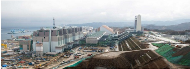
Figure 6. The 2200 MWe Green Power CFB plant in Samcheok, South Korea.
