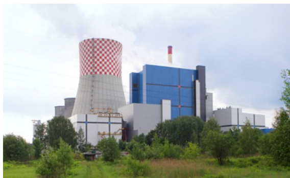
Figure 5. Lagisza CFB power plant, Bedzin, Poland. Source: Sumitomo SHI FW
