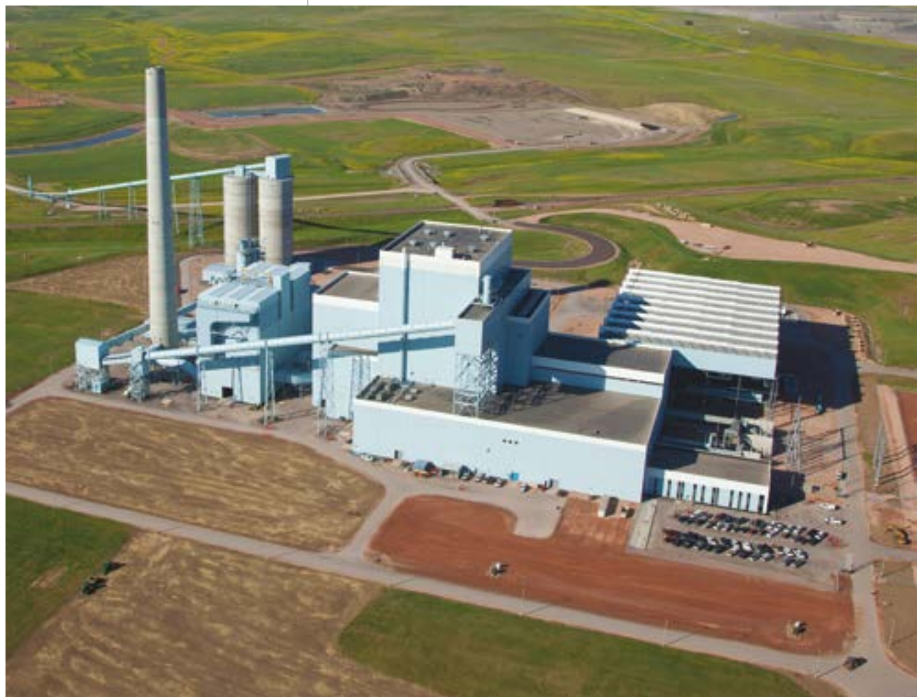
Right and below: Basin Electric Dry Fork Unit 1, with a plant electrical output of 420 MWe (or 520 MWe at sea level). The CFB scrubber at this plant, commissioned by SFW, is the largest in the world (photos courtesy Basin Electric Power Cooperative/ Wyoming Municipal Power Agency)
