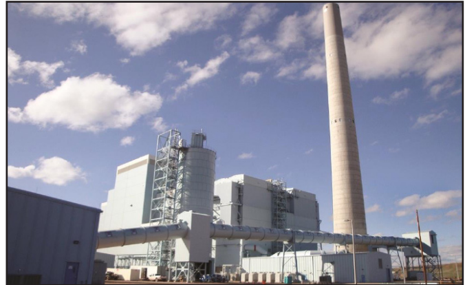
Figure 3. Basin Electric Dry Fork Unit 1 commissioned by SFW is the largest CFB scrubber in the world with a plant electrical output of 420 MWe or 520 MWe at SL (Courtesy Basin Electric Co-Op and Wyoming Municipal Power Agency)
