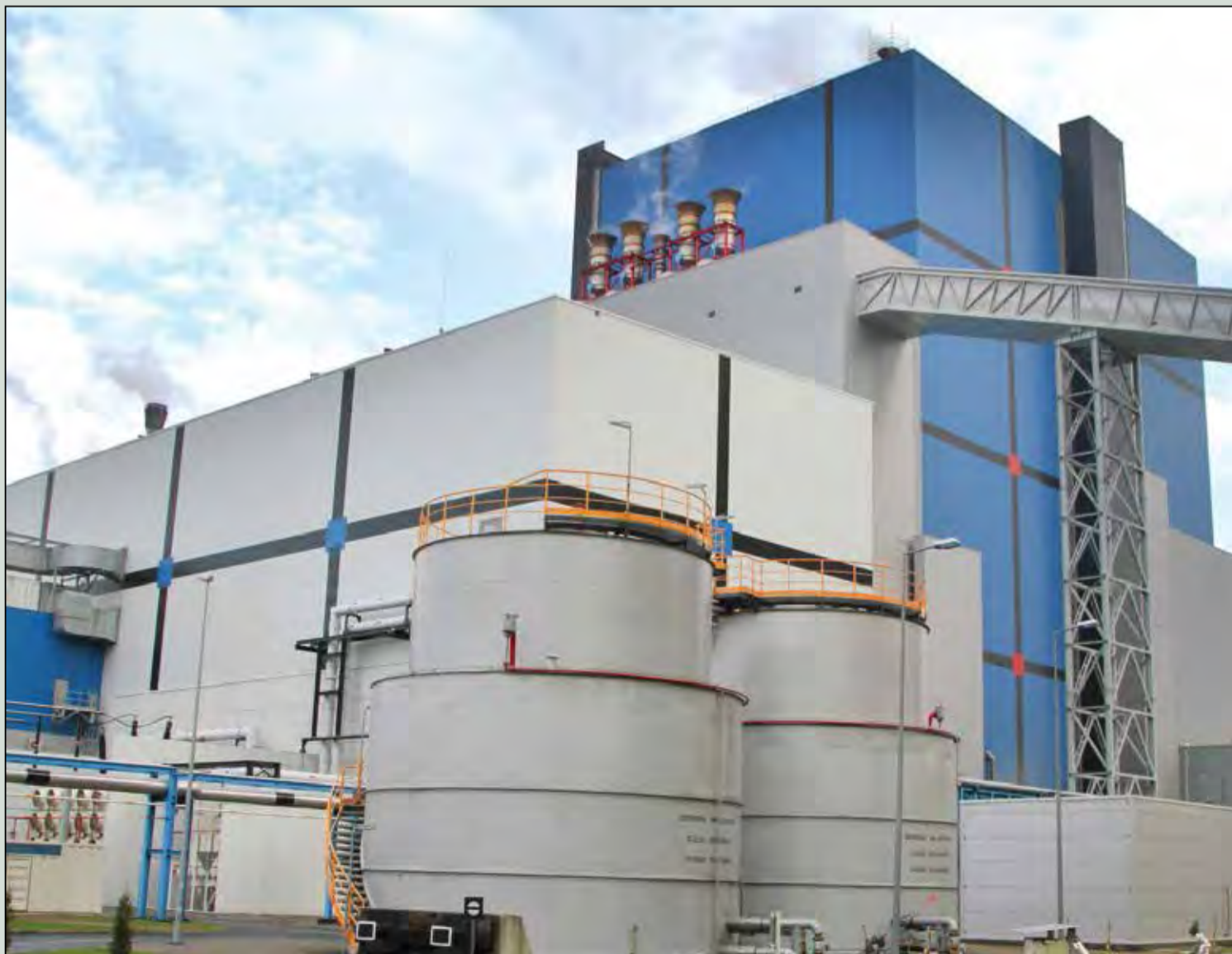
The technology advance to once-through supercritical (OTSC) units was first demonstrated at the 460 MWe Łagisza plant in Poland
